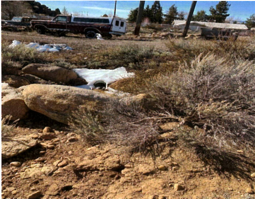
Photo 4. Inlet to culvert under Parcel A.
