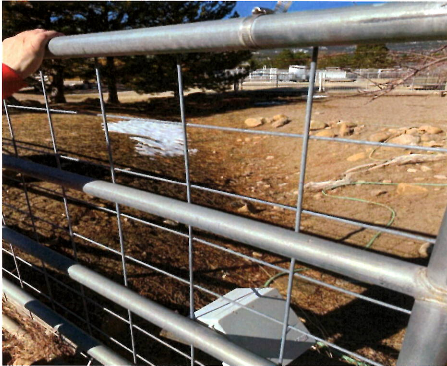
Photo 7. Outlet of culvert under Access Road.
