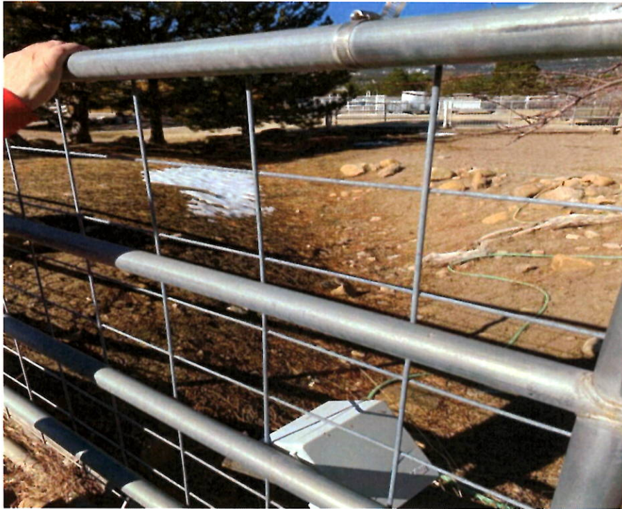
Photo 7. Outlet of culvert under Access Road.
