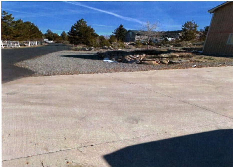
Photo 6. Looking north from Wolgast property to point at which flow is diverted west under Access Road.
