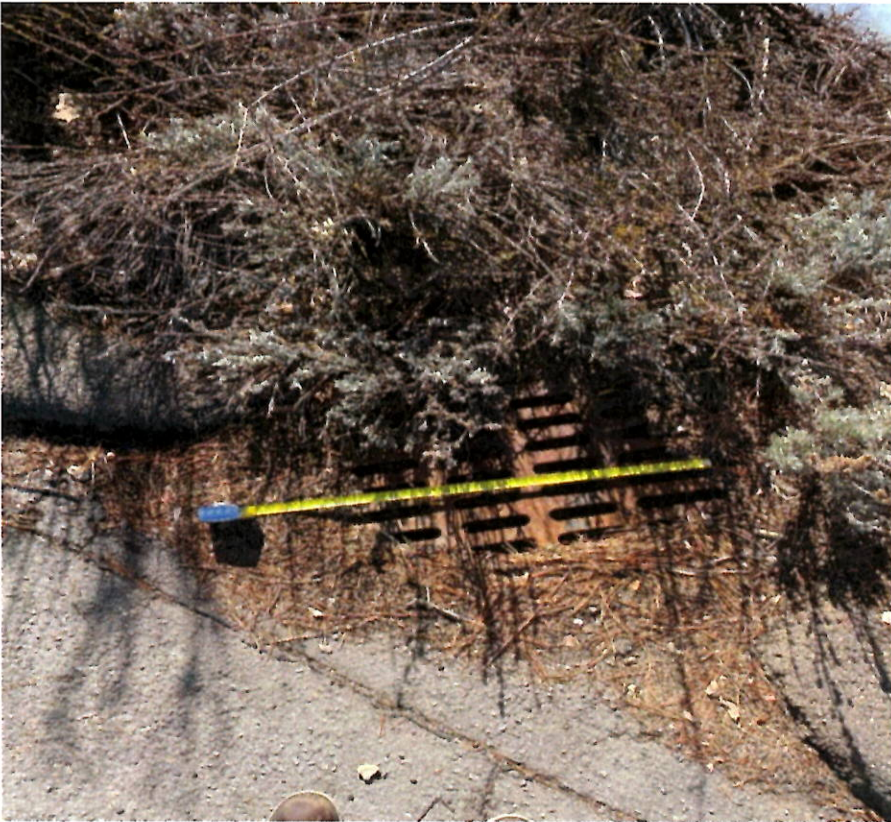
Photo 1. Storm drain on Cedarwood Drive near Access Road.
